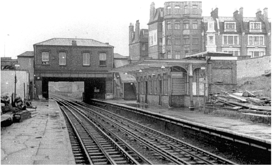
Above: At platform level looking east in 1968. The platform buildings are being demolished as part of the modernisation and rationalisation program for the line. The platform buildings had been repaired and rebuilt in about 1950 after suffering some minor bomb damage during the war. ( Photo: Jim Connor )
